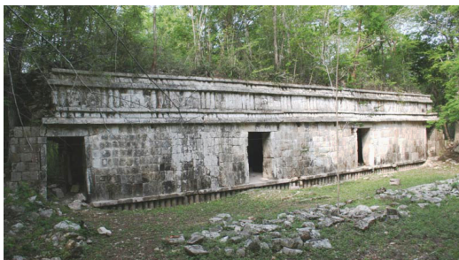
Figure 1: Photograph of a well preserved Puuc-style building in Kiuic, Mexico.
